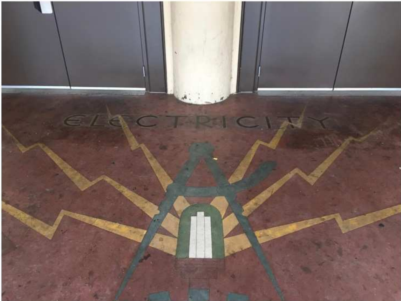
Clean existing entrance floor to Municipal Gym.
